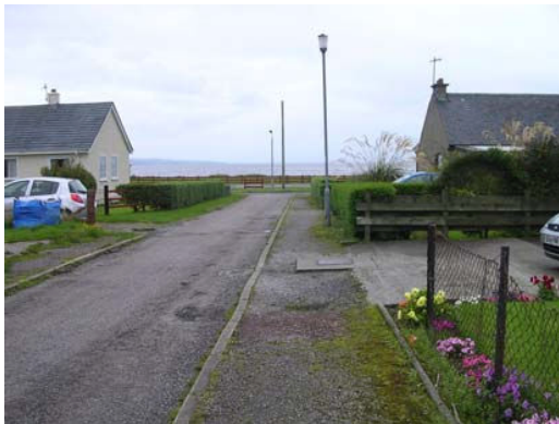
Sealand Housing Scheme Road
