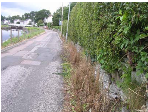
West Bank Road
